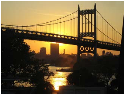
Building material for the Triborough Bridge
