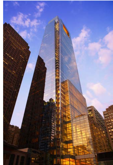
Construction material for the Comcast Building
